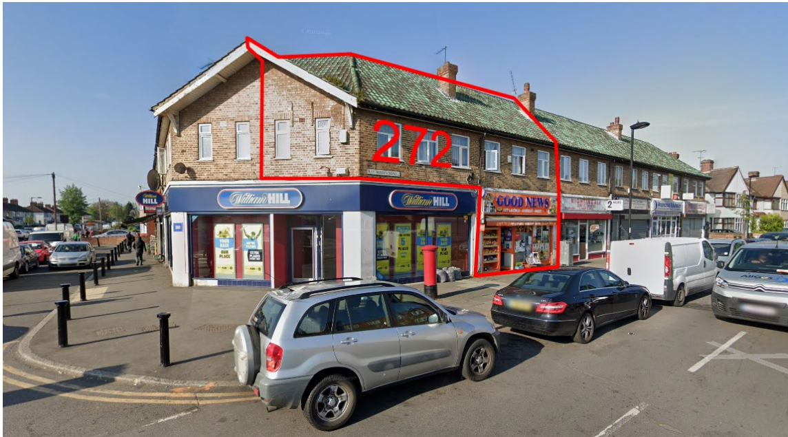
Image 1: Front elevation of 272 St Marys Road, as outlined in red
